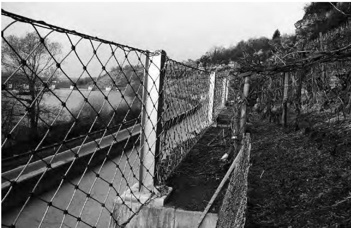
**Bildtafel 2: Steinschlagsicherung am Otto- Konz- Weg (2004)**
